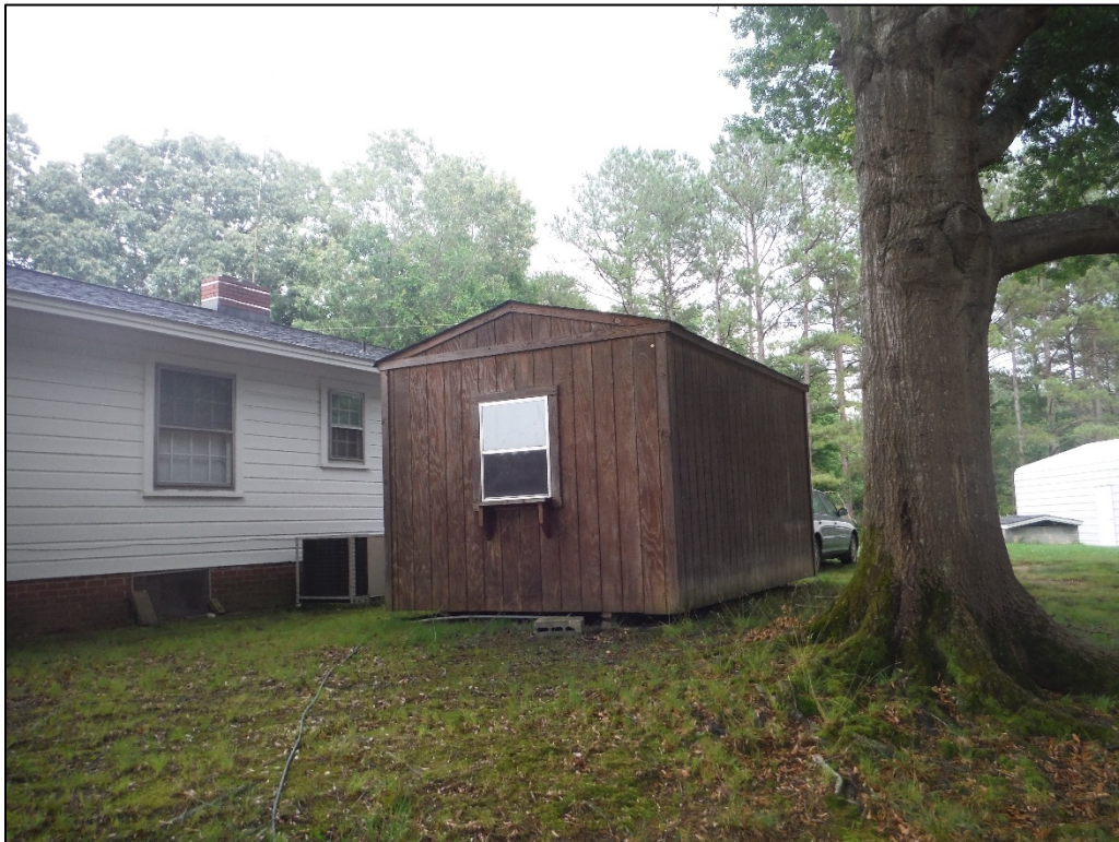
Figure 16. View of the late-twentieth century shed on the Freemon & Marie Cash House property, facing east.
