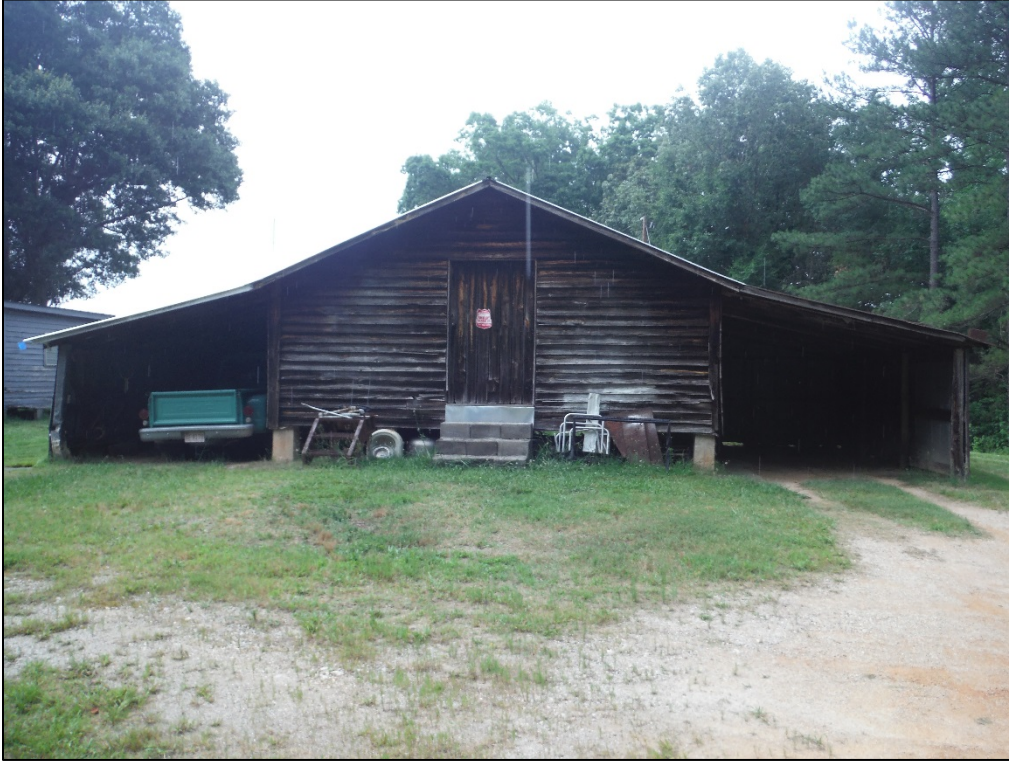
Figure 19. View of the mid-twentieth century granary on the Freemon & Marie Cash House property, facing north.
