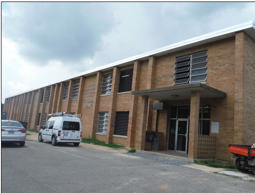
Figure 27. View of the T. J. Ellison Water Treatment Facility, facing northwest.
