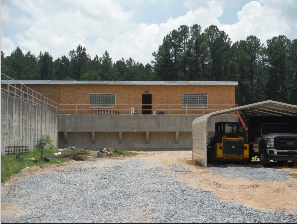
Figure 35. View of the office and treatment building at the T. J. Ellison Water Treatment Facility, rear elevation, facing south.
