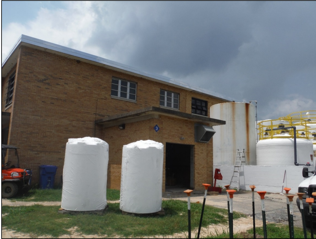
Figure 33. View of the office and treatment building at the T. J. Ellison Water Treatment Facility, east elevation, facing northwest.
