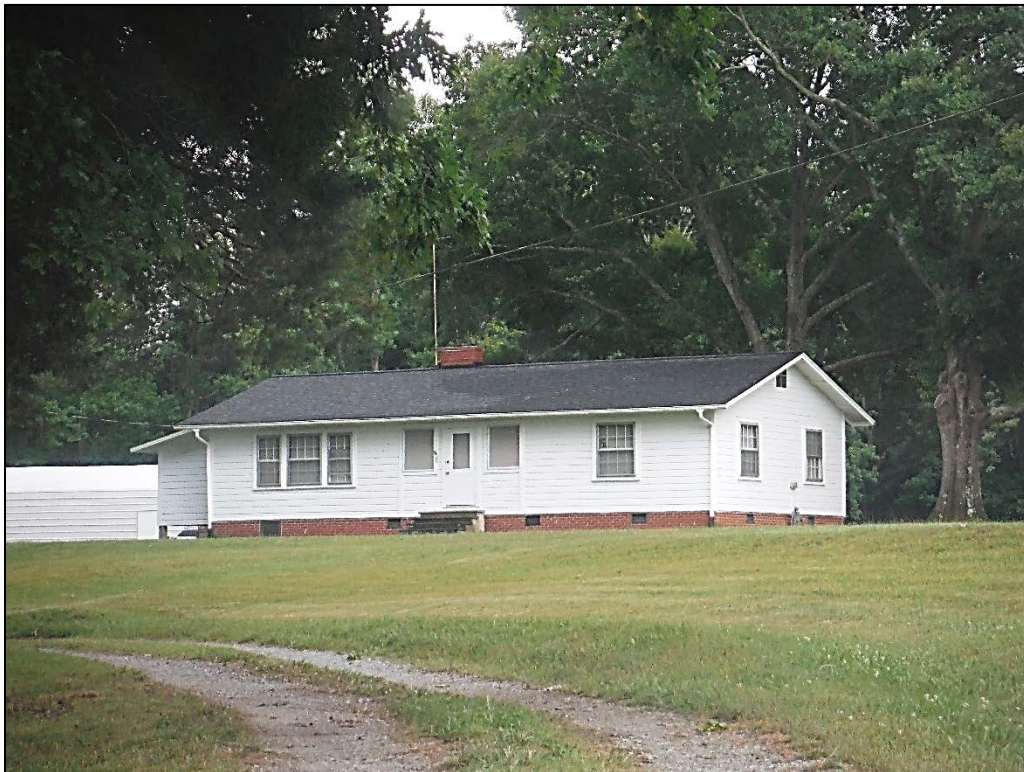
Figure 8. View of the Freemon & Marie Cash House, facing south.
