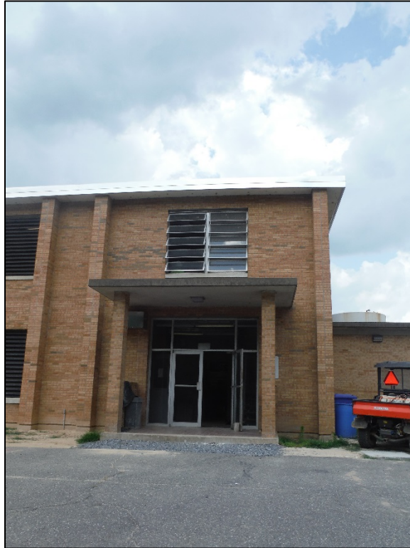
Figure 29. View of the entry bay of the T. J. Ellison Water Treatment Facility, facing north.
