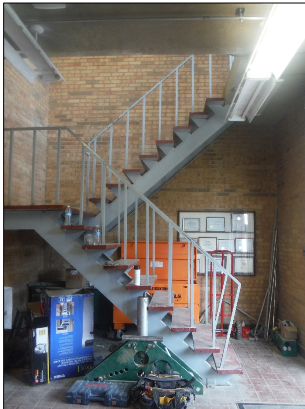
Figure 39. View of the interior stairwell of the office and treatment building at the T. J. Ellison Water Treatment Facility.
