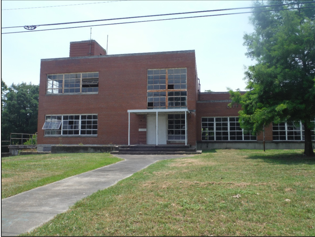
Figure 60. Lumberton Water Treatment Plant (RB0653), facing west.
