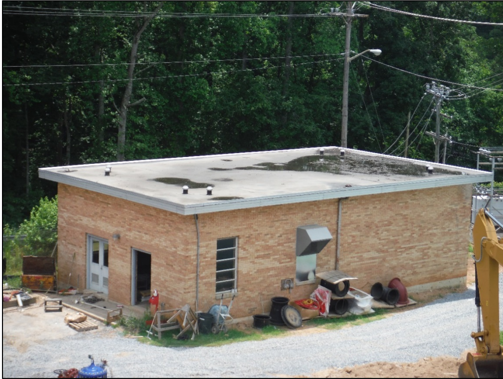
Figure 53. View of the pump building at the T. J. Ellison Water Treatment Facility, facing southwest.
