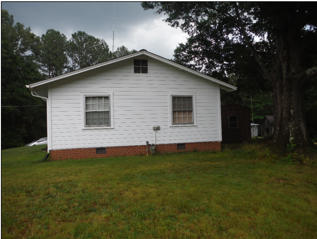
Figure 11. View of the Freemon & Marie Cash House, facing east.
