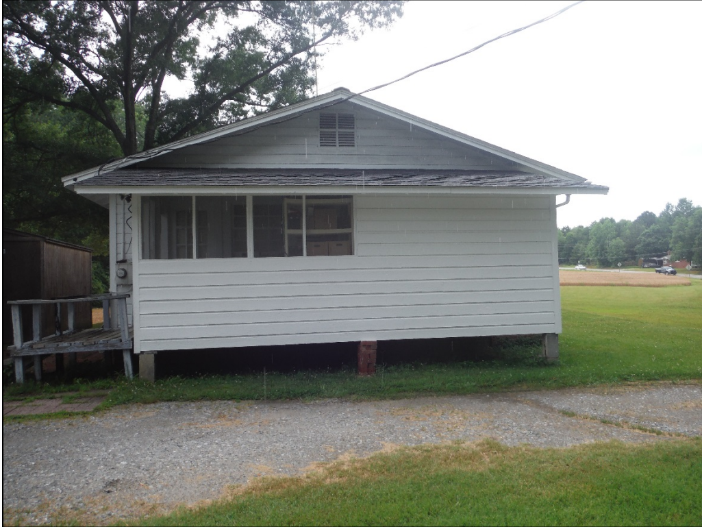
Figure 14. View of the Freemon & Marie Cash House, facing northwest.
