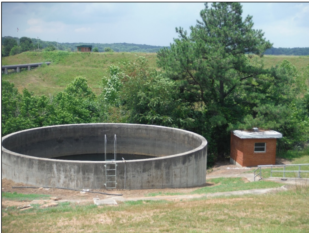
Figure 50. View of one holding tank at the T. J. Ellison Water Treatment Facility, facing west.
