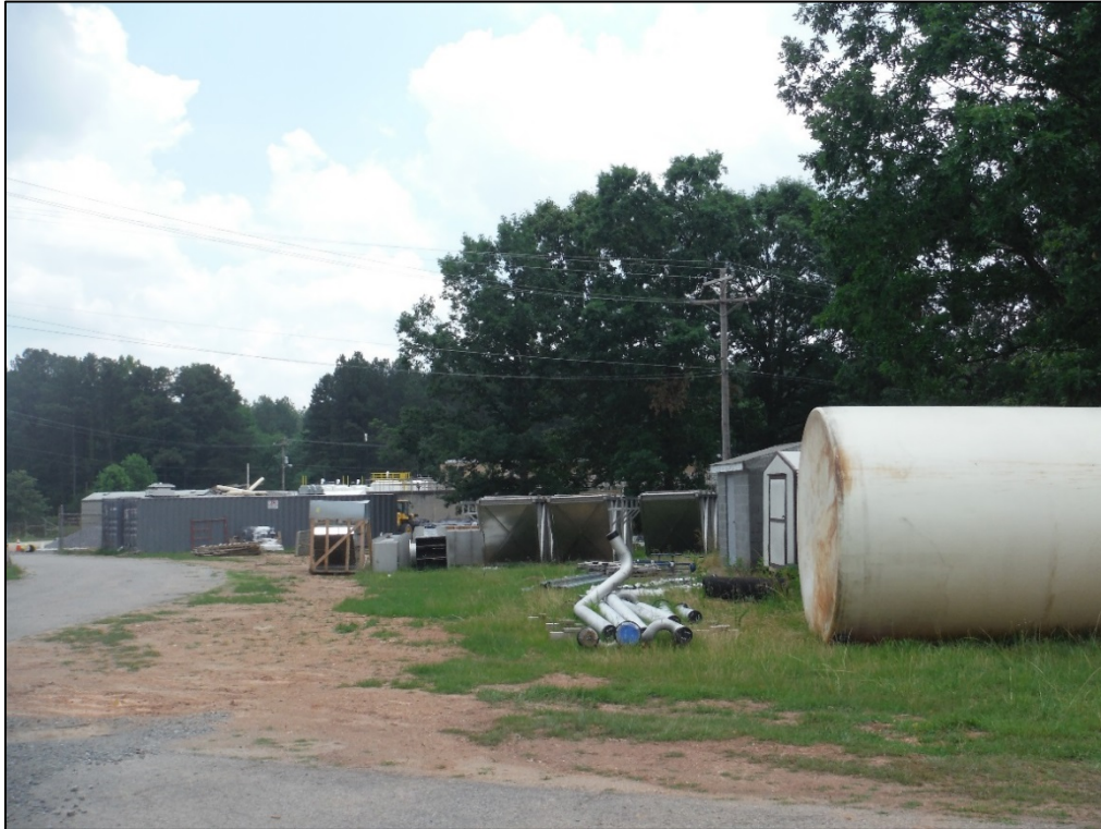
Figure 49. View of the storage and construction trailers behind the T. J. Ellison Water Treatment Facility, facing west.
