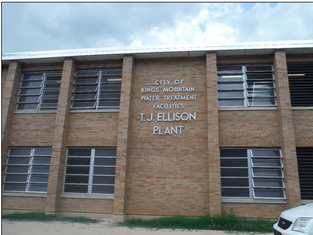
Figure 30. View of the front elevation of the T. J. Ellison Water Treatment Facility, facing north.
