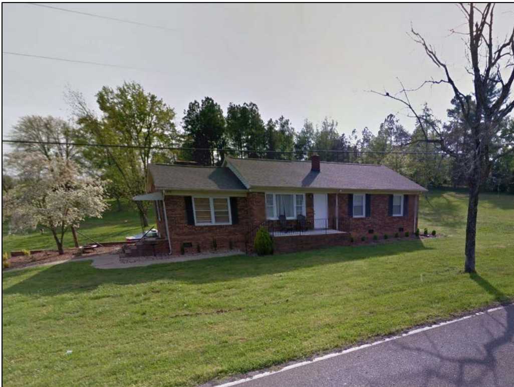
Figure 26. House at 2450 Oak Grove Road, facing northwest.
