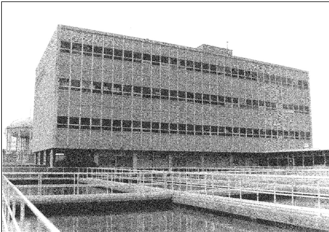
Figure 59. Franklin Water Works (MK2158).
