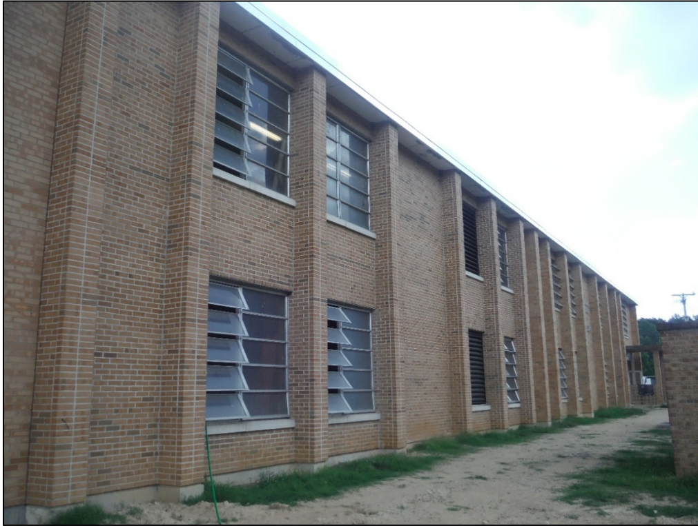
Figure 31. View of the office and treatment building at the T. J. Ellison Water Treatment Facility, facing northeast.
