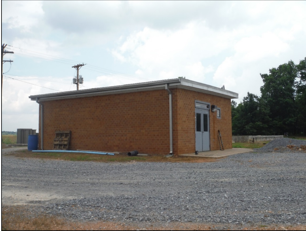
Figure 55. View of the sludge building at the T. J. Ellison Water Treatment Facility, facing northwest.
