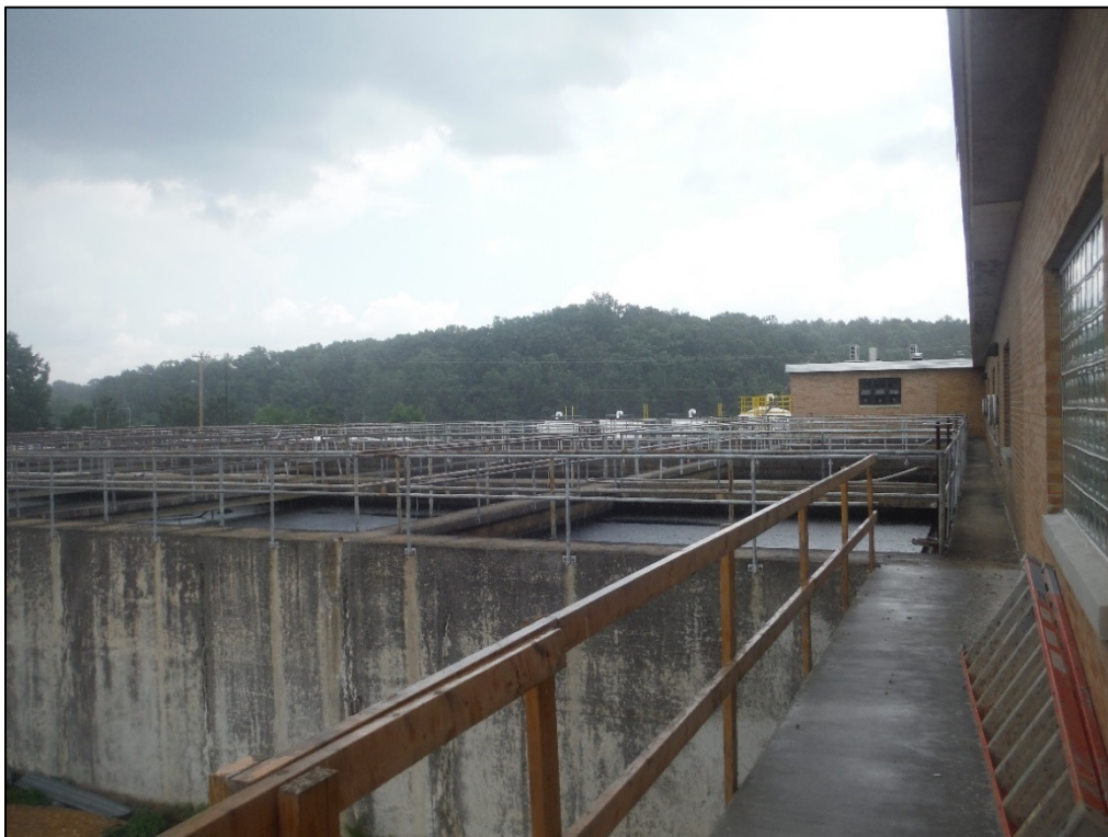
Figure 38. View of the office and treatment building at the T. J. Ellison Water Treatment Facility, basins at rear elevation, facing east.
