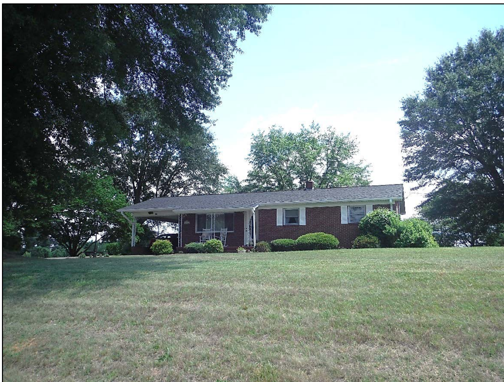
Figure 24. House at 2551 Oak Grove Road, facing east.
