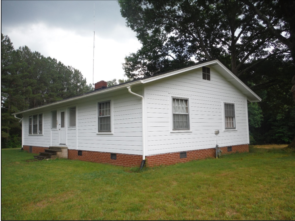
Figure 10. View of the Freemon & Marie Cash House, facing southeast.
