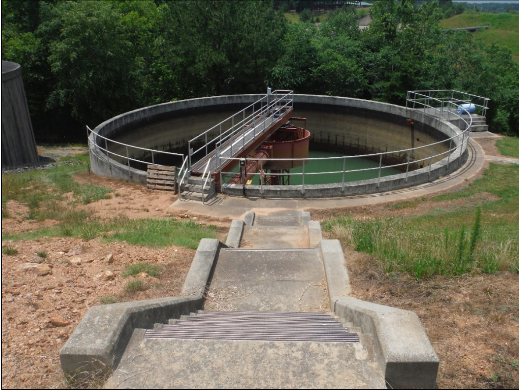
Figure 51. View of one holding tank at the T. J. Ellison Water Treatment Facility, facing west.
