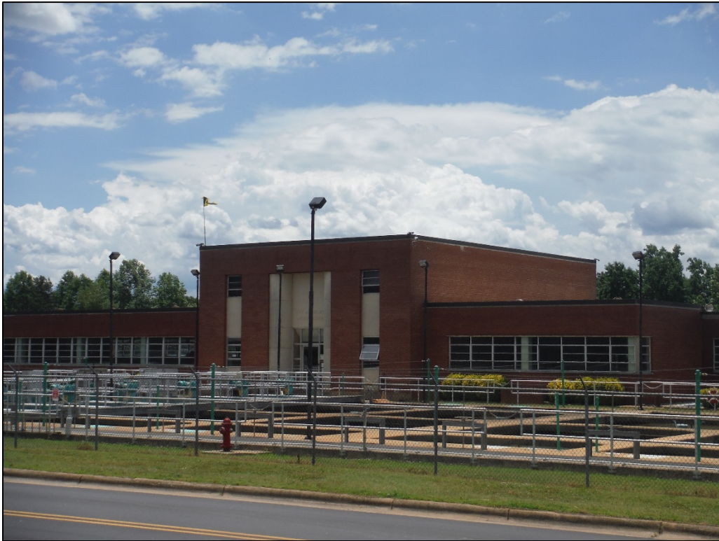
Figure 61. Shelby Water Works (CL0530), facing south.
